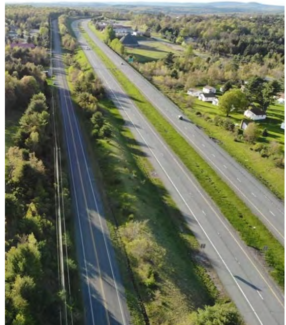
View along NY-17/I-86 looking northwest between Monticello and Harris.
