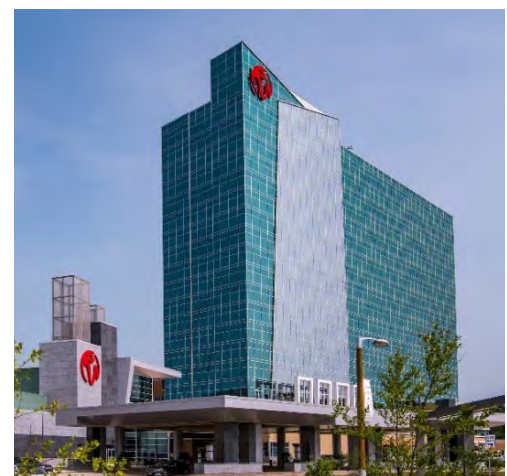
Resorts World Catskills opened in 2018 and features 65,000 square feet of gaming space and an 18-story hotel tower with 332 suites. It is a major economic driver and employs more than 1,000 people.
