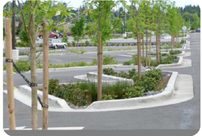
Examples of green infrastructure integrated into parking lot design. Green infrastructure allows for natural stormwater management by collecting runoff in permeable landscaped areas.
